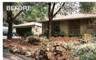
top and opposite Bill and Edie Dagley’s expanded master suite provides a more interesting street facade. New landscaping softens the end of the house. Inside, the dormer windows emphasize the bedroom’s new height.
